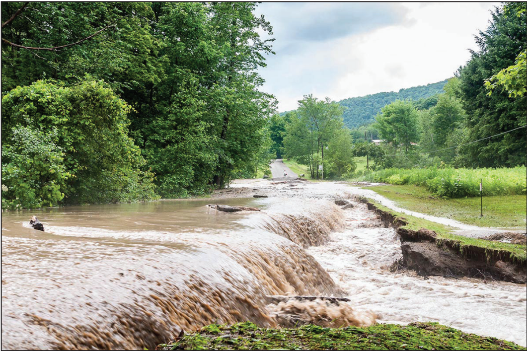
Texas Brook, usually a demure stream, overflowed its culvert and changed course across Texas Hill Road, Huntington on July 11.
