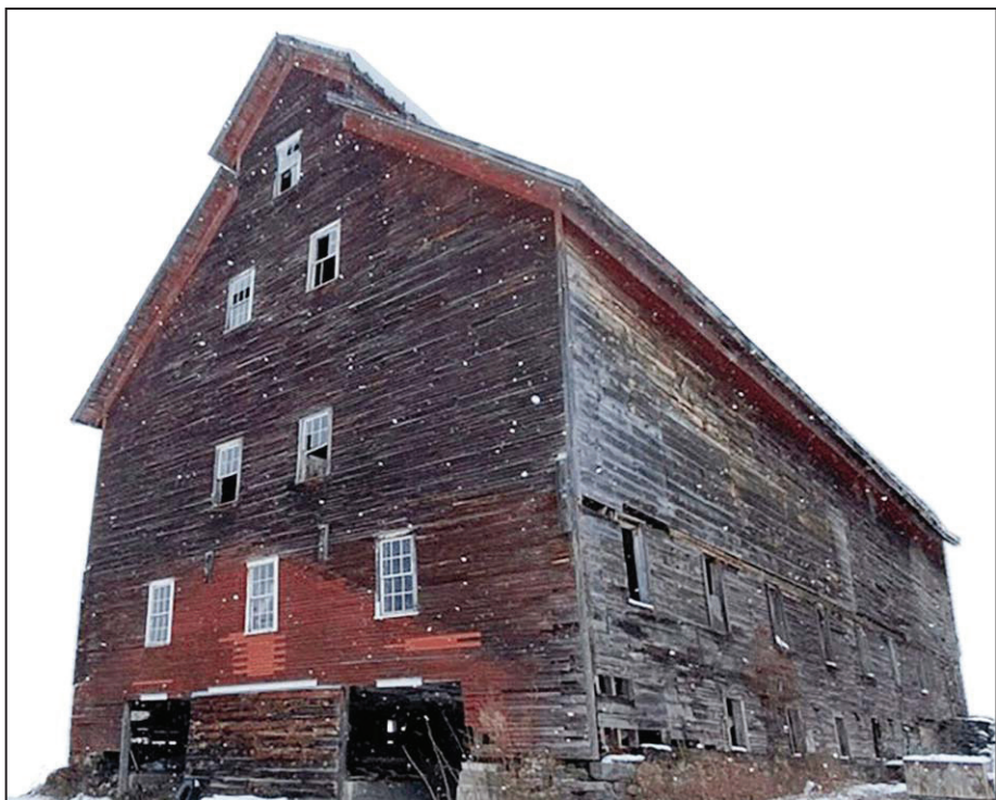
East Monitor Barn before restoration began in 2023. Courtesy photo
