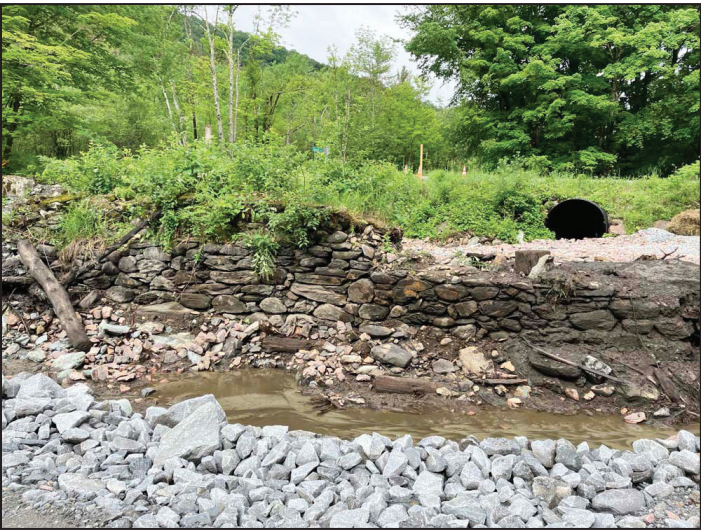
After 120 or more years of steadfast service, Gillette Pond's stone dam is history. Contractors removed it on June 11 to make way for a new and much stronger one. The Richmond Land Trust, owner of the Pond, expects the dam to be finished this summer – the capstone of a $1.1 million fundraising project. (Bob Low photo)
