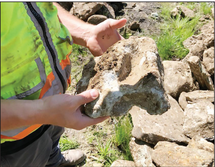
Crews discovered one reason the old dam shrugged off floods and ice jams for well over a century – its builders used concrete, too. Richmond's Jane Dorney, a consulting geographer who looks at how Vermont's cultural landscape patterns relate to the natural landscape, confirmed that "Concrete was used in some building projects in the early 20th century, although many refinements were made later." (Bob Low photo)
