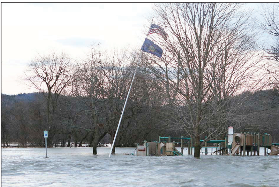
Richmond photographer Jared Katz spent the day on the edge of the climbing waters in the park in Richmond village on December 19. He captured the steady collapse of the newly repaired sign and flag base, which was necessitated by the July flood, and the height of the water that reached the top of the ladder on the slide (right side of photo) cresting near the top of the hill where the bandstand is located.
