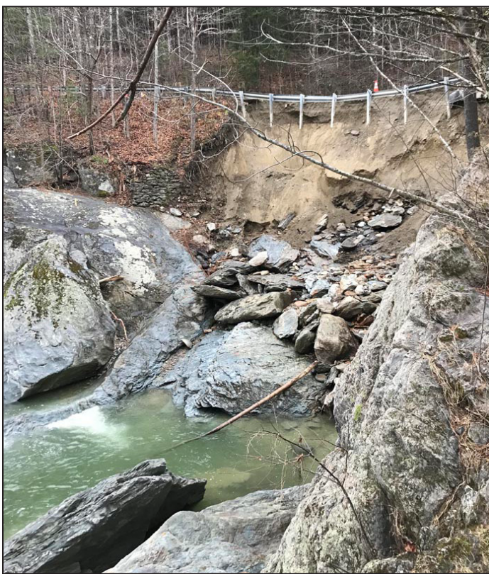
Above and left: flood damage to Dugway Road near the Huntington Gorge in Richmond has caused officials to predict that the instability will mean the road is closed to traffic for at least two months. Photos: Town of Richmond
