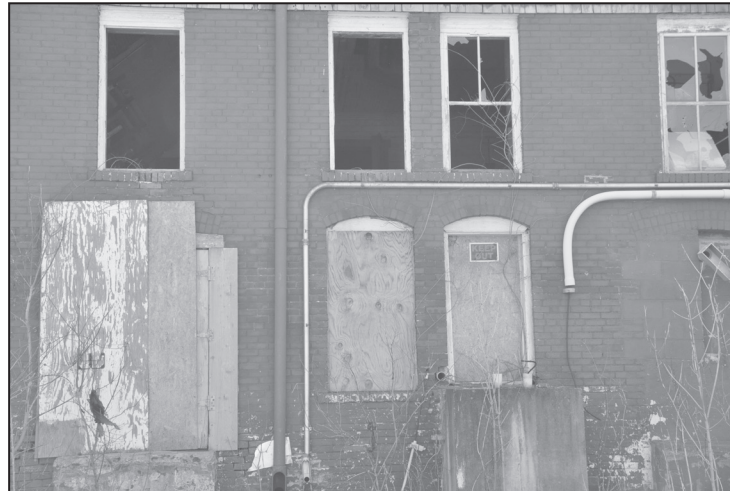
Not a single window is intact on the backside of one of the buildings at the dormant Richmond Creamery. Town officials have long worried about the safety hazards posed by the decaying structures. Photo: Greg Elias
