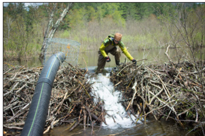
Vermont Fish & Wildlife technician Tyler Brown installs a water control device, or beaver baffle, on a beaver dam in Bolton. The baffle controls water levels to eliminate damage to a nearby road while maintaining the wetland for beavers and other wild plants and animals.
