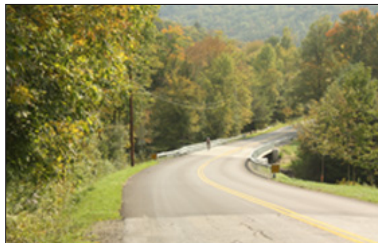
The narrow bridge on Huntington's Main Road north of Hanksville was replaced this summer. Extensive work required a detour, closed to large trucks. The site of accidents and one fatality in the past 30 years, the approach was straightened at both ends, making the bridge safer for all vehicles and cyclists. Photo: Heidi Racht
