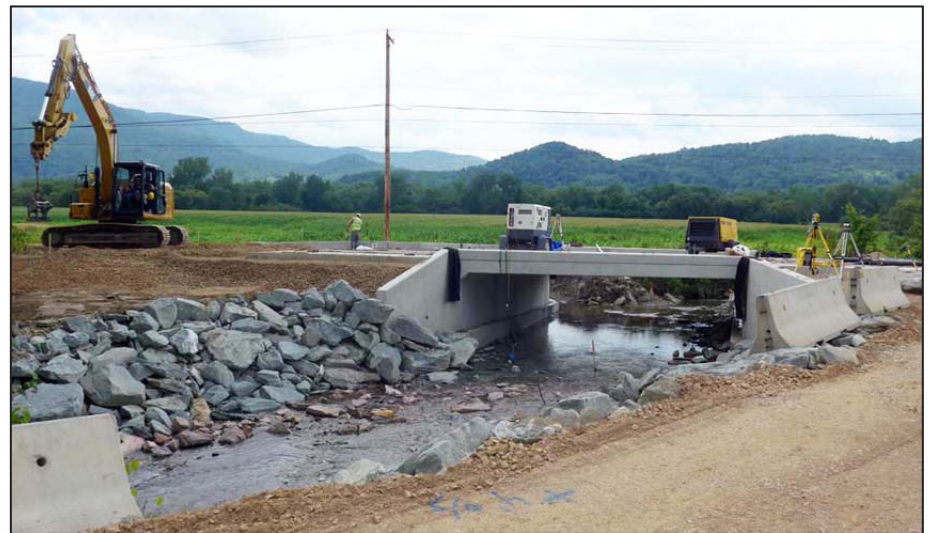
Above, anyone remember when Route-2 was concrete? Removal of the asphalt shows the old concrete road underneath. Below, bridge nearing completion.
